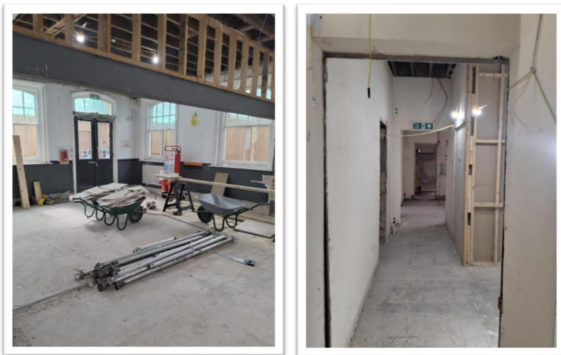
Left to right: The main corridor (old station building) and old ticket office facing entrance (old station building)
